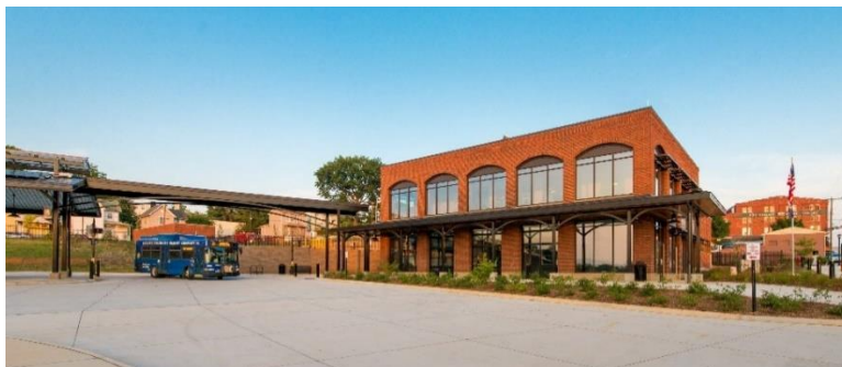
Figure 1-17: GLTC Transfer Station
